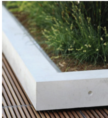
Figure 14. Exposed concrete plant bed
