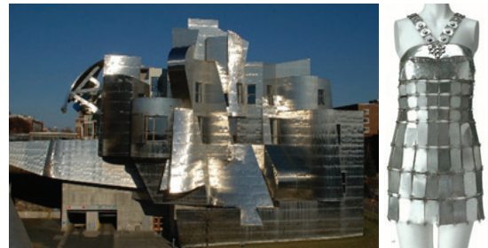
Photograph No 29. Weisman Art Museum, Frank O. Gehry ,2010. Photograph No 30. Paco Rabanne- Dress - 1967
