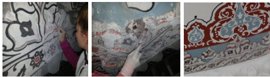
Image 15-16-17: Repair of the gypsum pieces, and the final version (From architect Fakir Cavlun)
